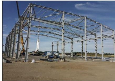
Figure 1 Erection of the NTS building primary structure (summer 2017)
