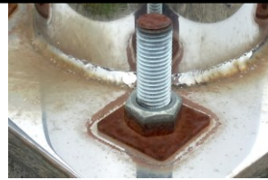
Galvanised steel fasteners on mirror-polished stainless steel
